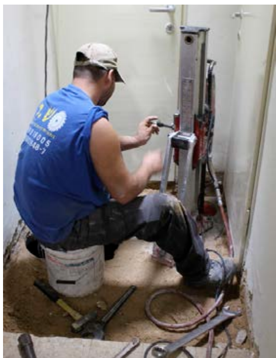
Figure 11. Drilling probe holes into the tomb
